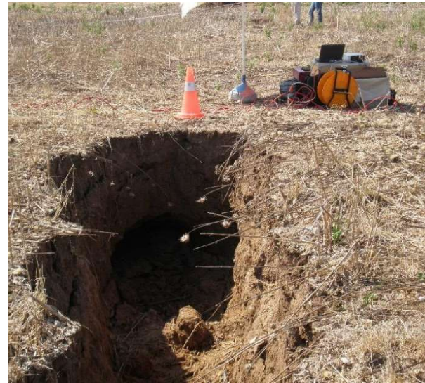
Figure 2: A ground fissure was identified in the field in close proximity to the village of Kileler.
