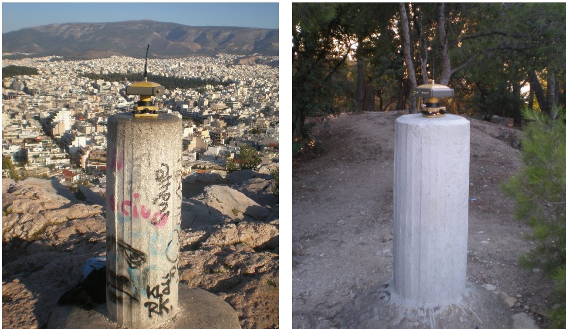
Figure 4.6: The Geodetic benches of the Hellenic Military Geographical Service of Filopappou (left) and Ardittos (right) that were used for the tie of the base of Thisseio .
