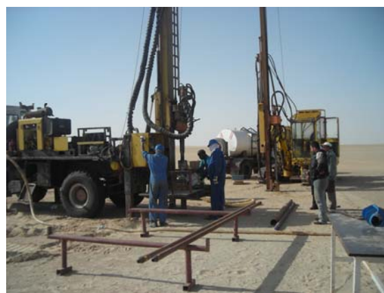
Figure 5. Drilling Boreholes 1 and 2 at As Sahabi, April, 2007
