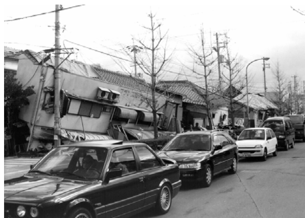
Figure 6. Destroyed wooden houses in Kobe.
