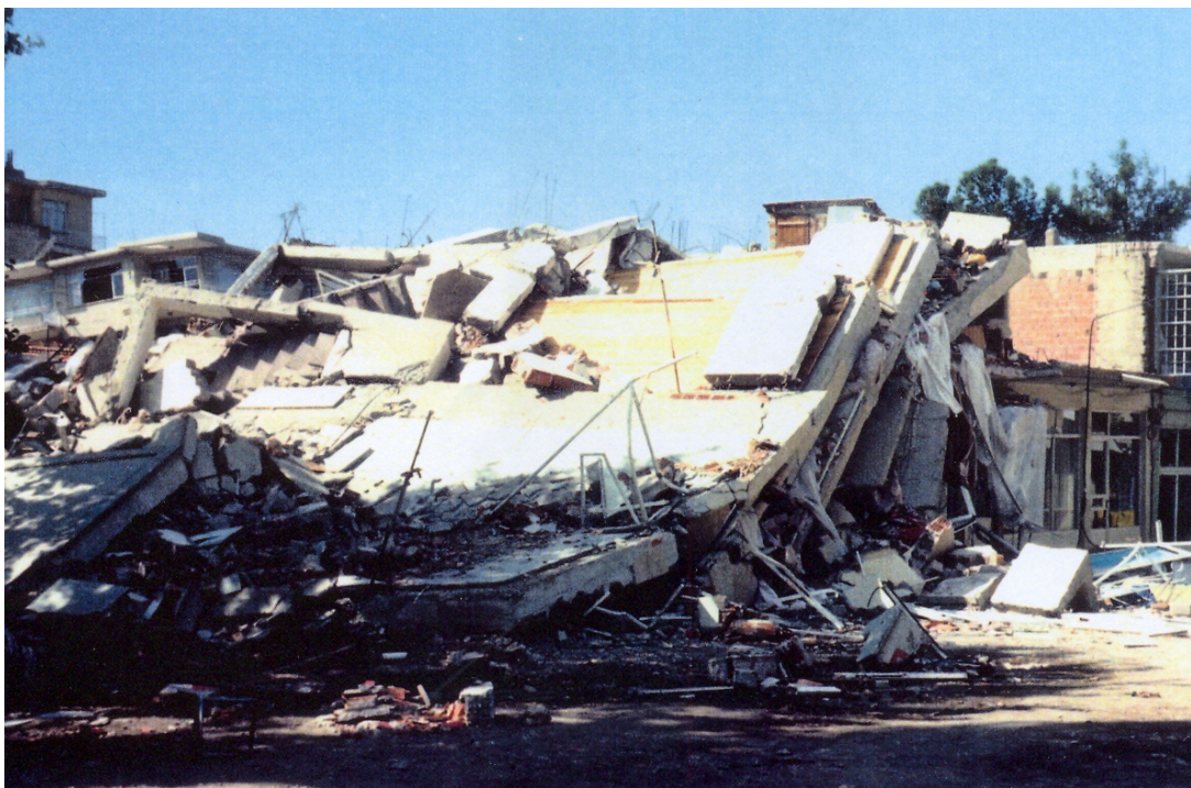
Figure 5. Collapsed multi-story residential building in Dinar.
