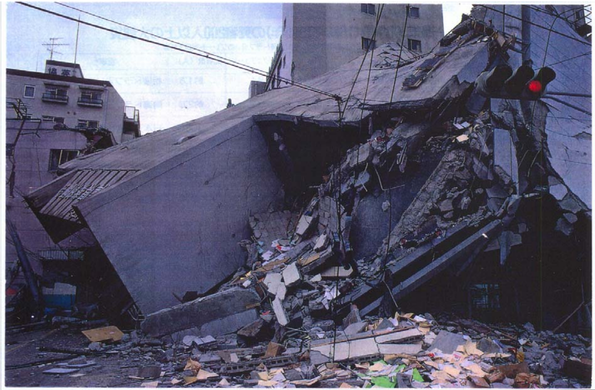
Figure 2. Collapse of a reinforced concrete building in downtown Kobe.
