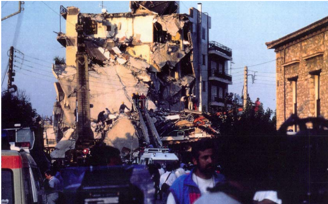
Figure 4. The collapsed apartment block in Egio, where 18 people were buried and died under it debris.
