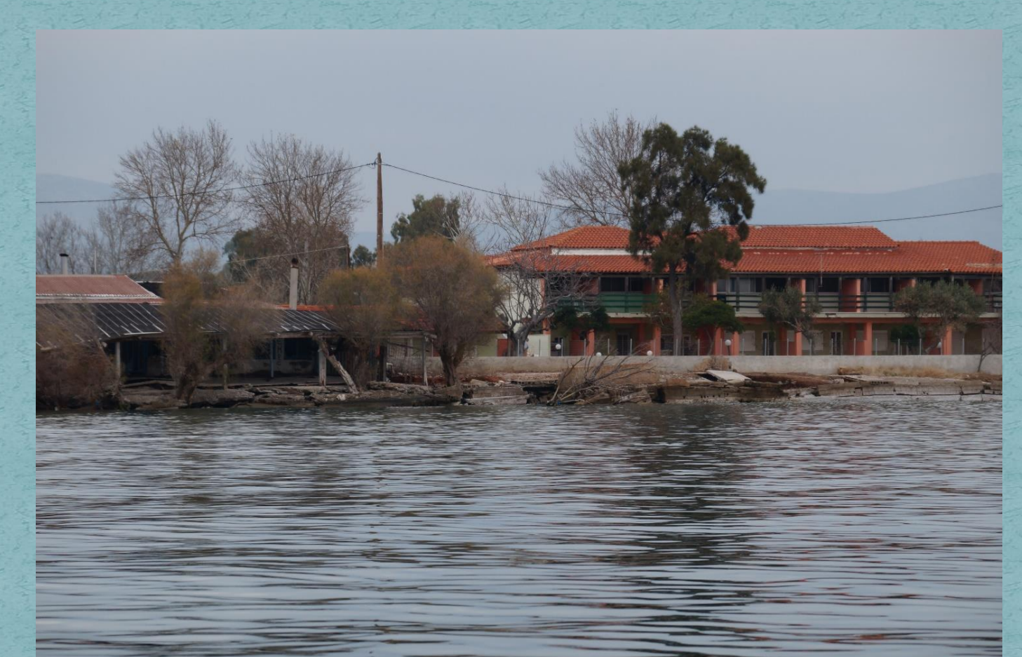
Figure 14. Destroyed restaurant by coastal erosion at Area 3 (estuary of Kenourgio stream)
