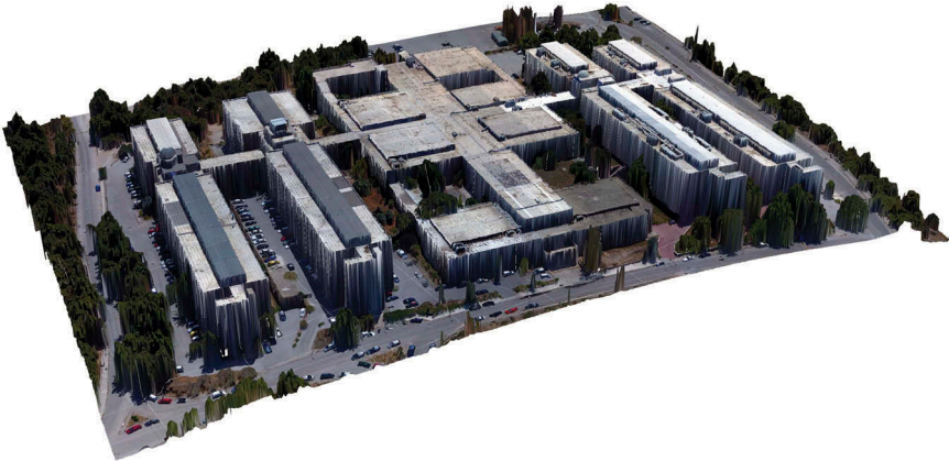
Figure 5. The combination of the high resolution elevation data and the ortho-image led to the construction of the high detail 3D model of the complex building area in the campus of National and Kapodistrian University of Athens.
