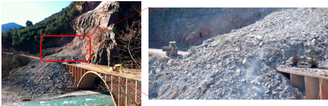
Figure 2. Archival photos from previous mass movement failures at the Proussos site (source: https://www.evritanika.gr ).
