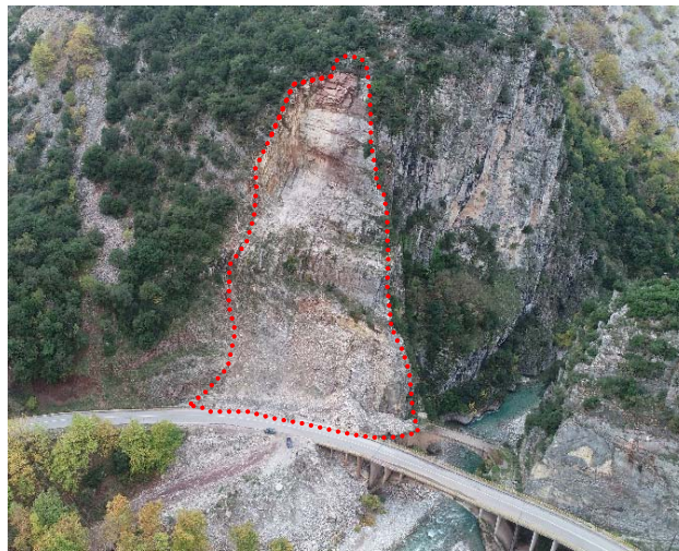
Figure 9. Aerial view from Proussos landslide site. Failure area is outlined with dashed red line.
