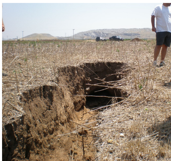
Figure 2 A ground fissure located in the field, close to village Kileler.
