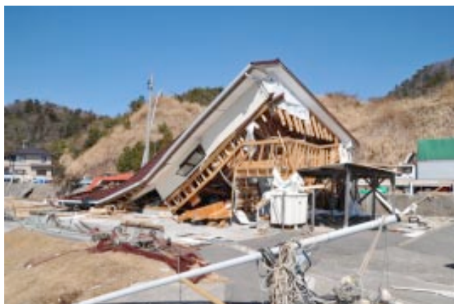
Fig.2. Collapse of a wood frame house in Iwaki area. Tsunami height of about 5 m
