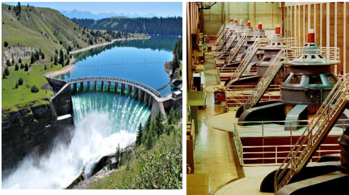
Figure 15. The 194-MW Kerr Dam in Montana of USA. The giant generators at Hoover Dam that produce on average, about 4 billion kilowatt-hours each year for use in Nevada, Arizona, and California - enough to serve electricity for 1.3 million people.
