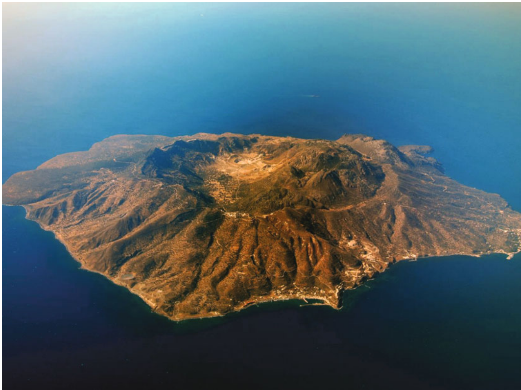
Fig. 3.2 Aerial view of Nisyros volcano from northeast; the caldera with an approximate diameter of 3.6 km the filling of the western part with voluminous rhyodacitic domes up to 698 m (Profitis Ilias); the almost circular
